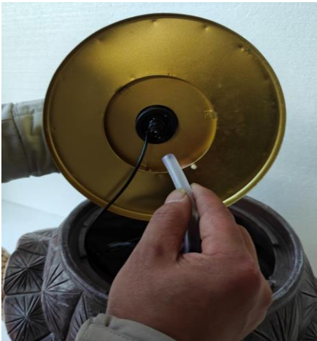
Attach the tubing from the pump to the corresponding connection from the top part of the fountain.
