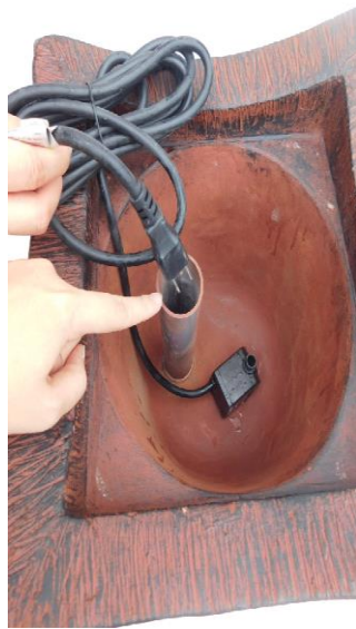
Pass the power cord of the pump down the cord pipe.
