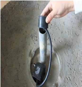
Install the cord pipe cover over the cord pipe as shown.
