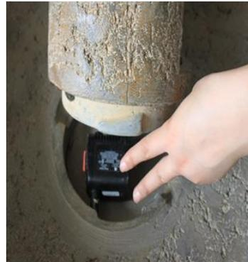
Set the riser in to place, align the grooves then twist and lock it to the bowl.
