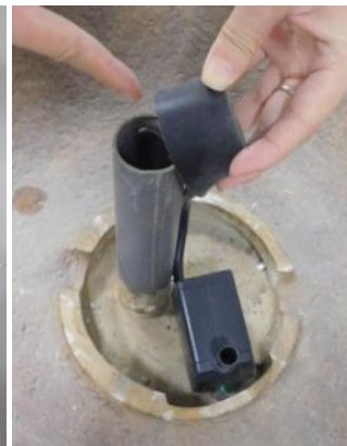
Install the cord pipe cover by aligning the cord then fitting it over the pipe and cord.
