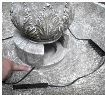
For discreet installation, the light cable can be passed through a water return location (above left) or through a location for accessing the pump (above right). Installation will vary based on the fountain.
