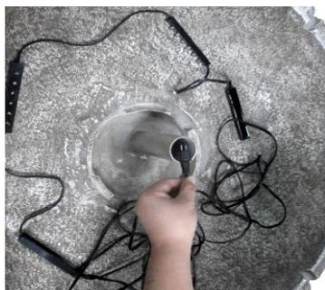
Position the lights in the desired location, then pass the power cable down the cord pipe or out the side of the fountain.
