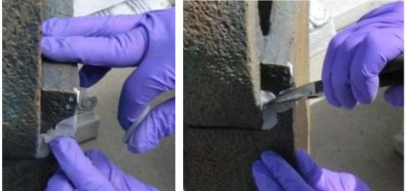
Apply putty to cover more than the affected area, pushing firmly around the edges to ensure a tight bond, and reduce the seams creating a less noticeable repair.
