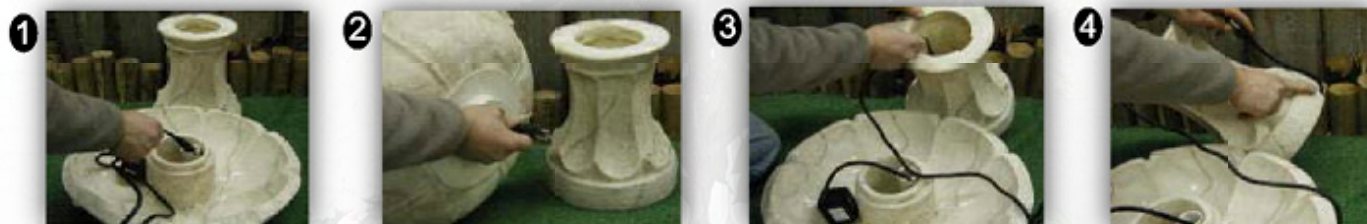
1-4 Start by passing the pump cord through the bottom bowl, then through base, setting into grooved notch at bottom.
