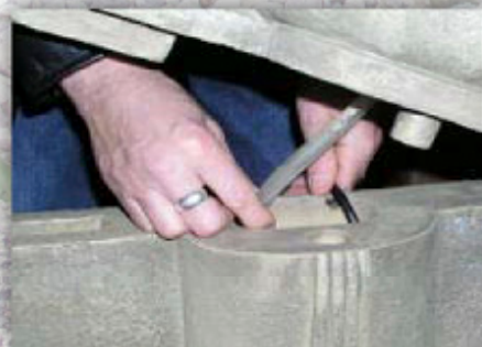
carefully lower pump into cavity, keeping cord in groove
