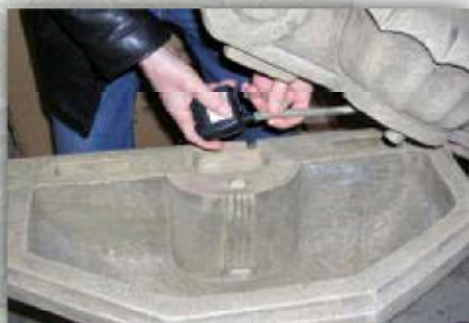
attach pump, check that tubing length allows pump to sit at bottom
