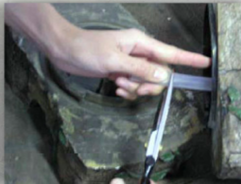
Measure the amount of tubing needed and cut excess to prevent bending
