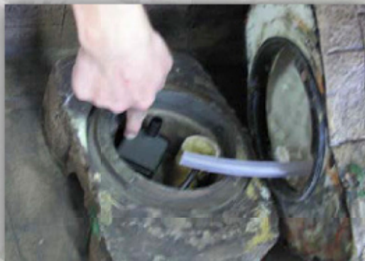
Measure the amount of tubing needed and cut excess to prevent bending
