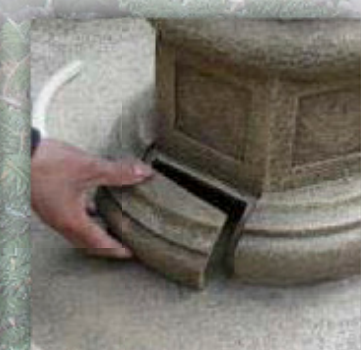
install access door
