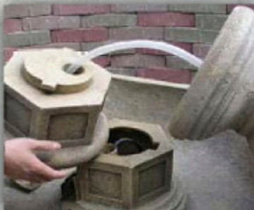
run tubing for pump through riser
