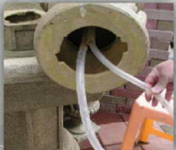
extra tube is for over flow pipe if desired
