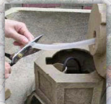
trim excess tubing so pump sits on bottom of bowl
