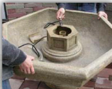
cord through pipe
