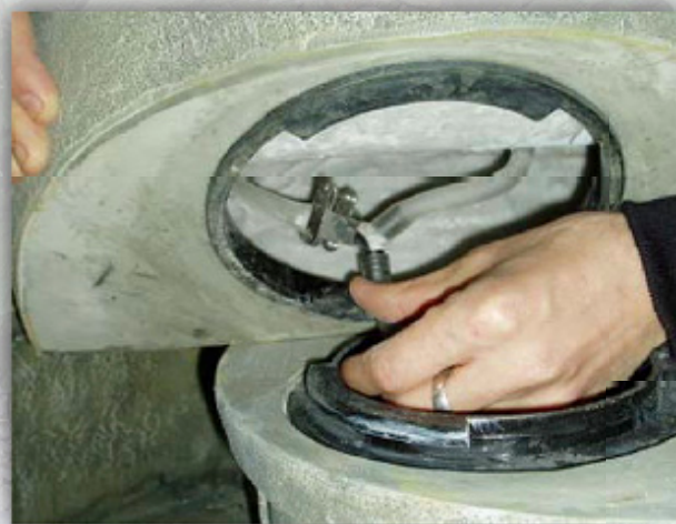
Note position of restrictor for water adjustment secure top to bowl using twist and lock
