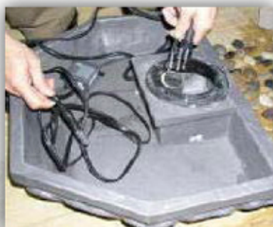
unplug light from transformer, run cords through pipe
