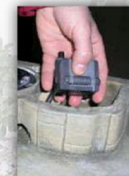
adjust pump to 1/2 strength
