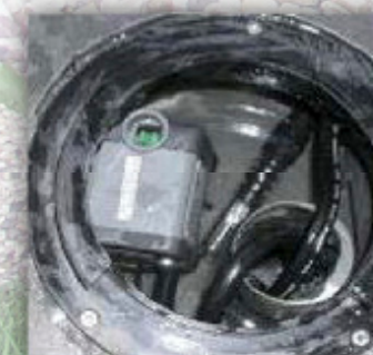
This is how pump and light should be positioned to insure efficient lighting
