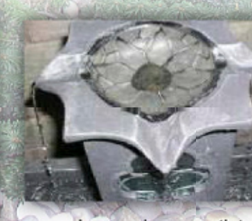
place rock over outlet to achieve a smooth flow
