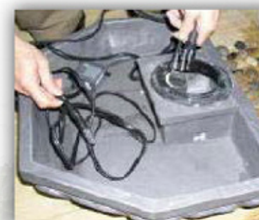
unplug light from transformer, run cords through pipe
