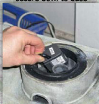
place pump in cavity
