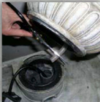
cut tubing to size
