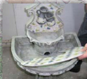
place pump in cavity
