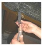
Connect the tubing from the feature using the copper connector.
