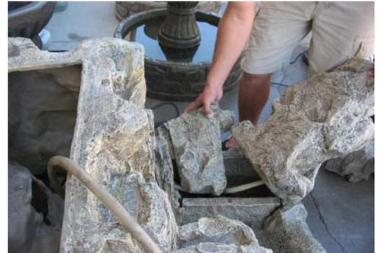
Once you have run the tubing and electrical chords install the side and top cover pieces with section number 2 as illustrated.
