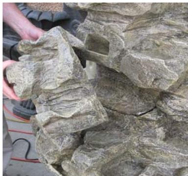
Attach section 4 to section 3 using groove as illustrated.
