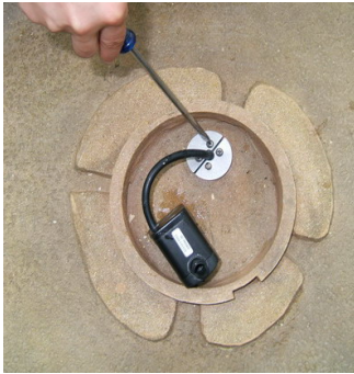
Ensure all of the screws on the pre-installed cord seal are tight.
