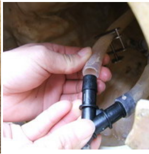
Using the included connection and "Y" joint, connect the tubing from the top sections as shown above.
