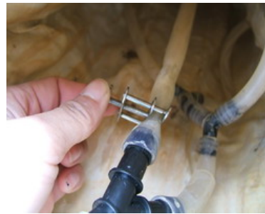
Adjust the restrictor as desired to increase or decrease water flow.
