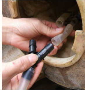
Using the included connection and "Y" joint, connect the tubing from the top sections as shown above.
