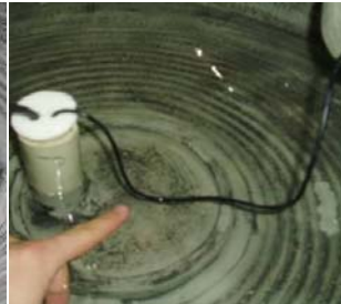
Securely install the rubber bung as shown. For the light cord, allow the cord to dip into the water before placing it down the cord pipe as shown above right. To reduce any chance of seepage, apply silicone along all seams of the rubber bung.
