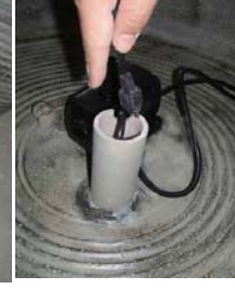
Light cord through pump cover, then through PVC pipe as shown.
