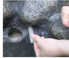
Pass the tubing down the opening (as shown above) and align with the hole to the main reservoir.
