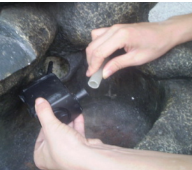
Connect the tubing to the pump.
