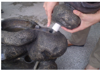
Slide the top into place by aligning the pipe and corresponding groove.
