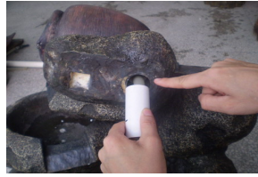
Pass the tubing through the "slip fit" pipe and install the pipe into the top feature as shown above.
