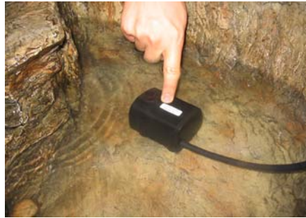
Place the pump inside the fountain as shown above.
