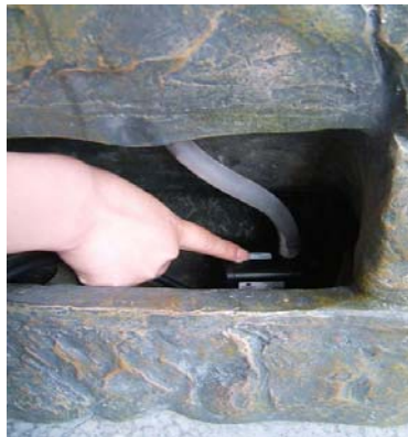
Pump should sit flat and move free inside pump house.
