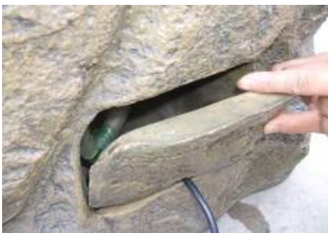
Install the pump access door.
