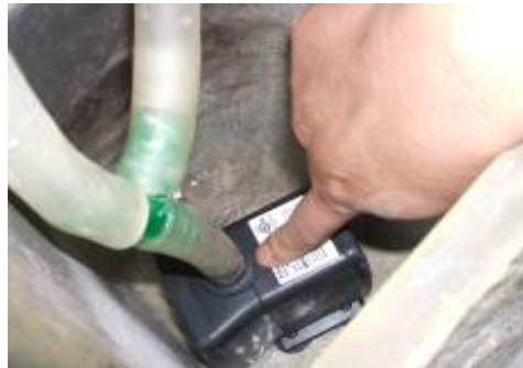
Set the pump securely in the base of the pump housing.
