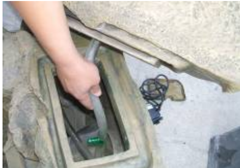
Place the tubing from the upper section inside the pump housing.
