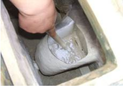
Place the tubing from the lower section inside the pump housing.
