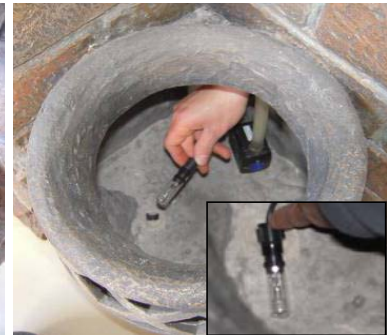
Pass the light in to the fountain from the rear access hole and press it in to the holder as shown above.
