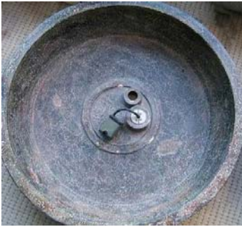
Pump comes pre-installed with cord seal. Check to see the cord seal is tight.
