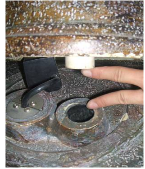
Set pump housing into place.
