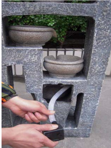
Locate the tubing from inside the fountain and connect it to the pump.
