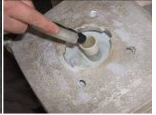
Run tubing and light cord from the orb, down the cord pipe.
