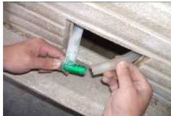
Connect the tubing to the "T", then connect the other end to the pump.
