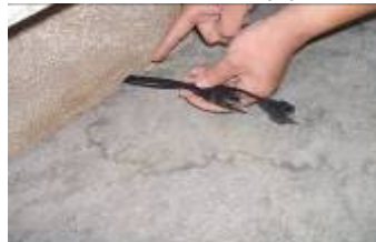
Feed the light cord through the cord pipe and align both cords with the groove at the base of the fountain.
