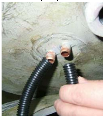
Connect tubing to the pump.
