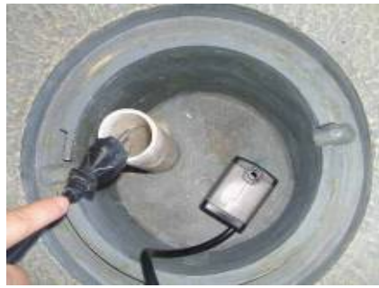
Pump cord through pedestal
