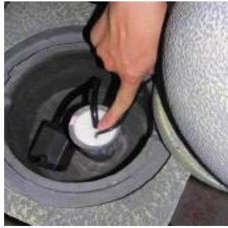
Make sure both power cord go through pvc pipe, lead to the groove at bottom. Insert rubber bung as shown.
