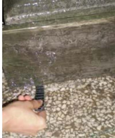
To achieve the maximum effect of this fountain, you will need to prepare the surface by rubbing the water into all areas when first starting the unit. You should also keep the unit as level as possible by using the shims we have included.
