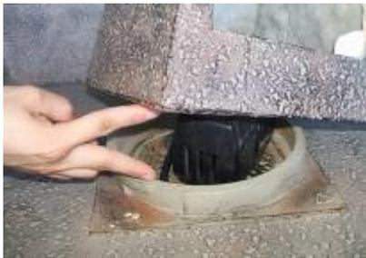
Twist and lock riser into place.
