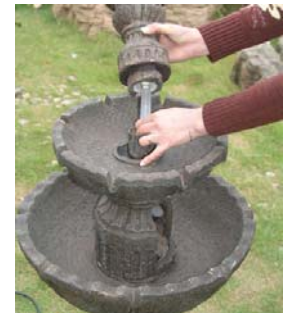
Connect the tubing to the top.
