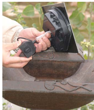
Connect the installed tubing to the pump.
