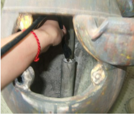
Feed the pump cord down the pipe.
