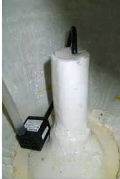
Install the pipe seal as shown above.
