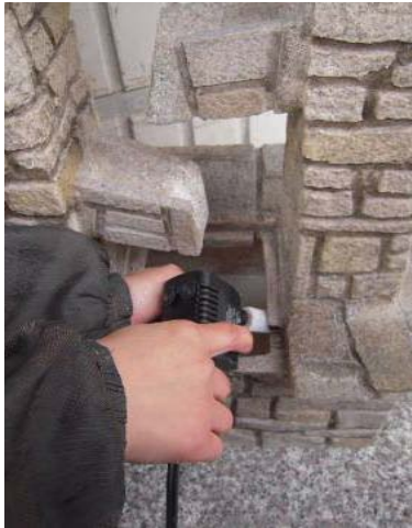
Locate the tubing from inside the fountain and connect it to the pump.
