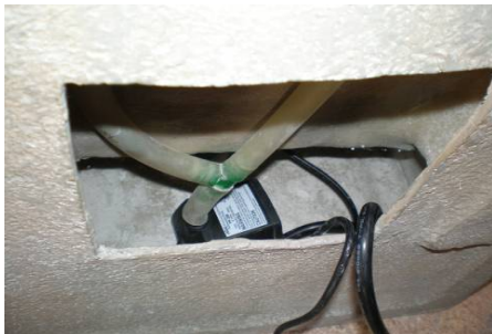
Set pump inside pump housing.
