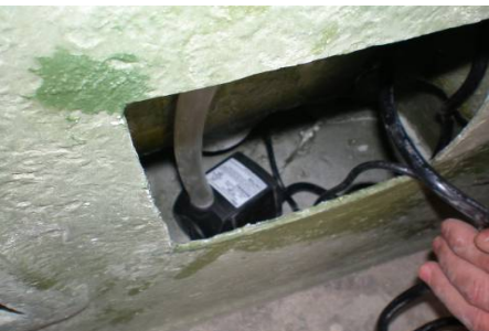
Set pump inside pump housing.
