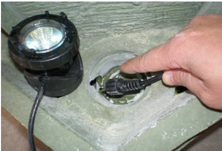
Feed the light cord through the hole, and out the access section at the back.
