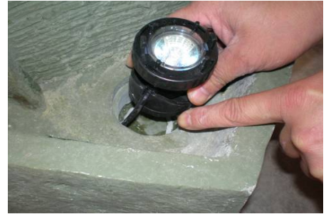
Set the light into place
