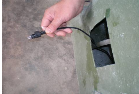
Feed the light cord through the hole, and out the access section at the back.
