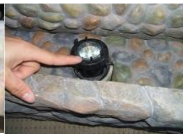
Set the light into the groove of cover plate and set the cover plate into place. Adjust the direction of light as desired.
