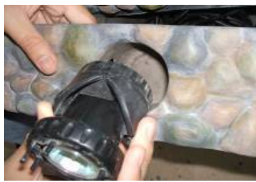
Set the light into the groove of cover plate and set the cover plate into place. Adjust the direction of light as desired.
