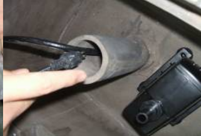
Run the light cord through the cover plate, then through PVC pipe.
