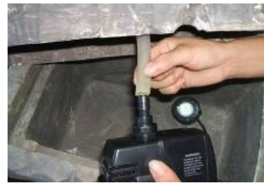
Run the light cord through the cover plate, then through PVC pipe.
