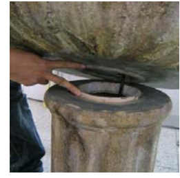
Twist and lock the bowl to pedestal.
