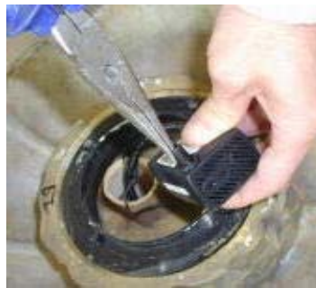
pull pump outlet out with pliers
