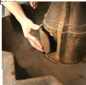
Install the pump access door.
