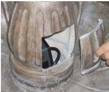
Install pump access door.
