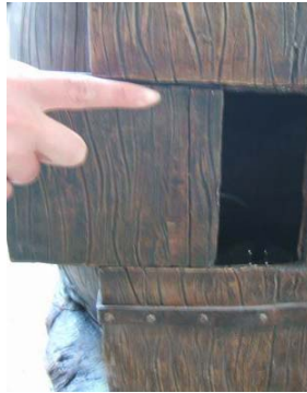
Install the pump access door.
