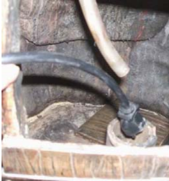
Cord through standpipe
