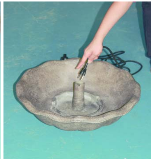
Pass the power cord down the cord pipe in the bowl.
