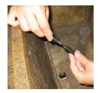
Feed 1 of the 2 light power supplies into the pump housing and through the center water return hole ash shown above right.
