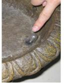
Next, take the other light fixture and feed the side which will connect to the power through the opening in the bowl of the top feature.
