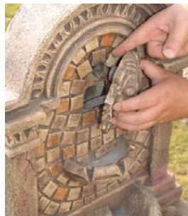
Once you have passed any excess tubing into the fountain, align and slide the feature face in to place.
