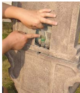
Connect the tubing from the feature to the opening output on the "T" connection at the rear of the fountain.
