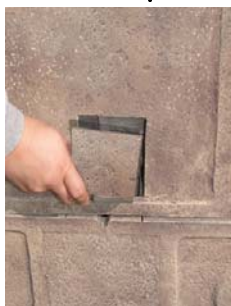
Install the access door.
