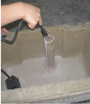
Pump cord through standpipe
