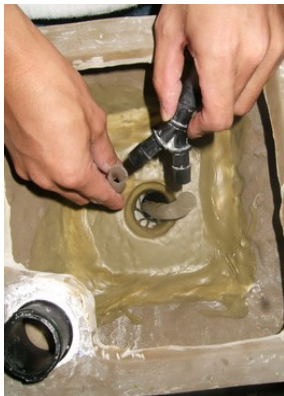
Connect tubing with T joint
