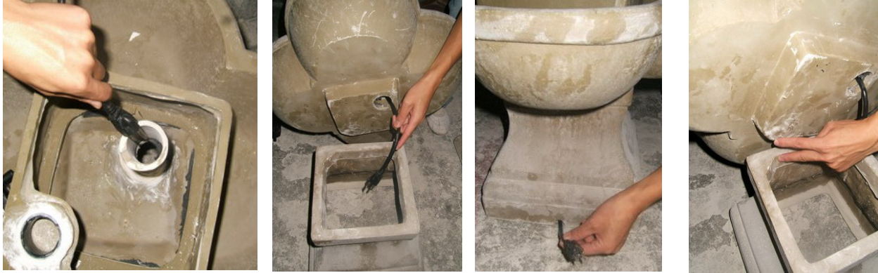
Pump cord through standpipe
