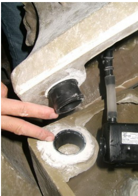
Connect tubing with T joint
