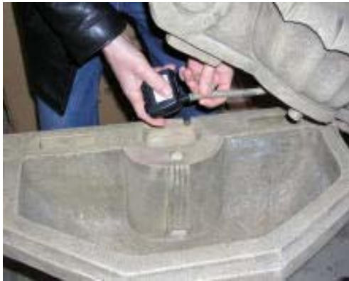
attach pump, check that tubing length allows pump to sit at bottom
