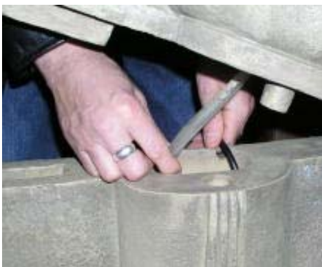
carefully lower pump into cavity, keeping cord in groove
