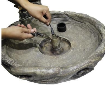
Pass the light cables down the cord pipe.
