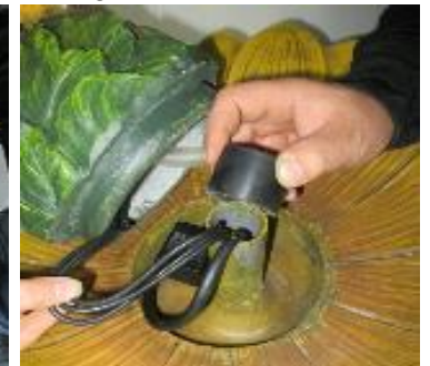
Install the cord pipe cover over the cord pipe and cords as shown.
